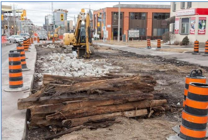
Work continues on **King, from Union to Wellington**, to accommodate the relocation and upgrading of underground utilities, such as watermain and stormwater.
